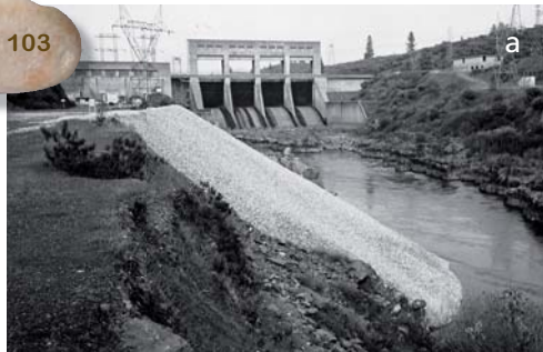
(a) transfert des alluvions en aval du barrage Keswick, Sacramento River, California (1997). (b) http://www.trrp.net/implementation/sediment_management.htm#cs
